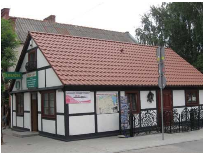
12. Timberframe building at Wiejska Street
