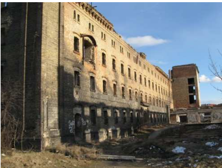
18. The former slaughterhouse has been repeatedly set on fire ...
