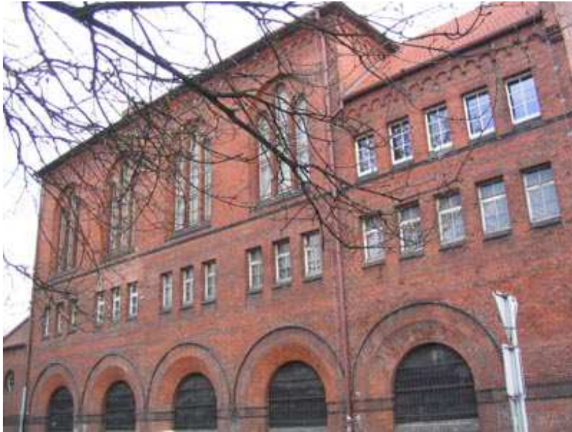
22. The building of the former bathhouse
