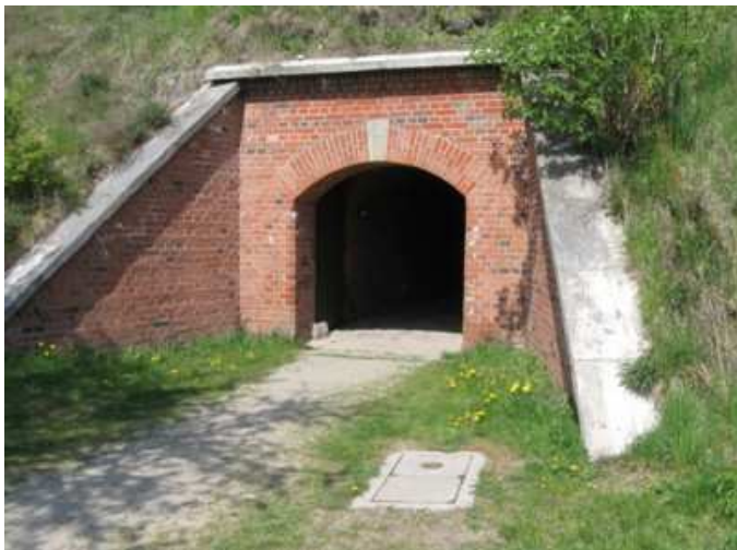
8. Fortifications were subjected extensive renovations works
