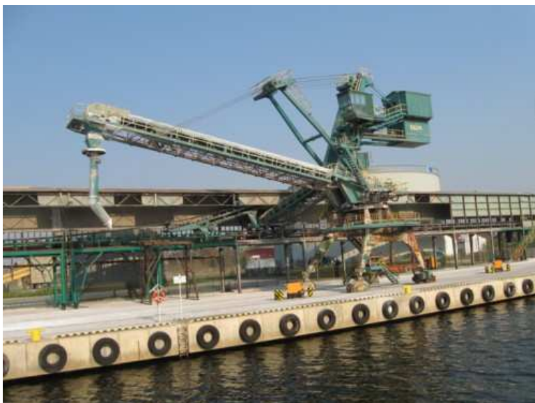
15. Loading quay in Gdansk Port
