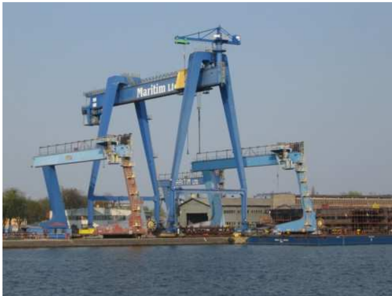
13. Maritim Shipyard infrastructure
