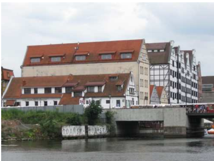
3. The Green Bridge
